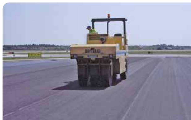
Compaction is often specified for airport jobs
